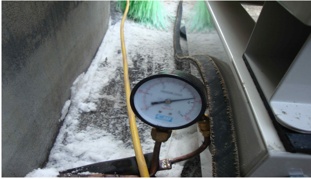
냉매배관 VACUUM TEST
