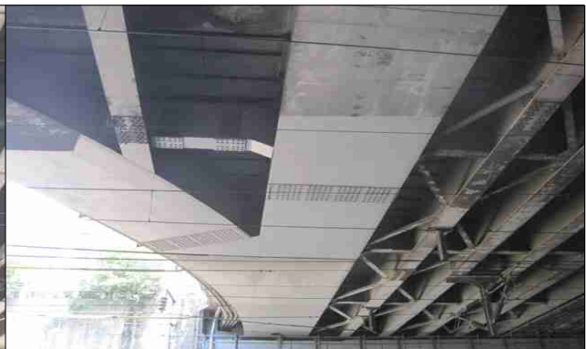
Steel Box Girder
