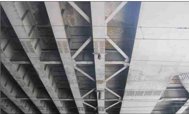
Steel Plate Girder
