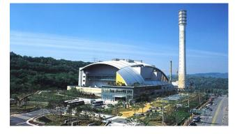
The facility was created in May 2005 after prolonged use of landfills for the northwest region of Seoul. It has the capacity of incineration for 750 tons of waste per day (250 tons per day × 3 units). The wastes are safely incinerated at high temperatures. Recycled
