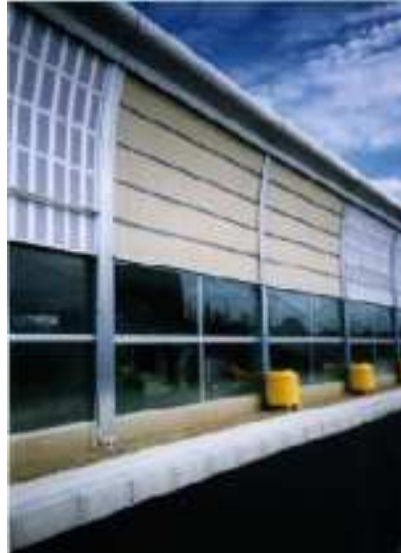
#302 National road Nagoya city
